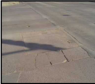
Overlay & Concrete Pavement Restoration $40.7M
